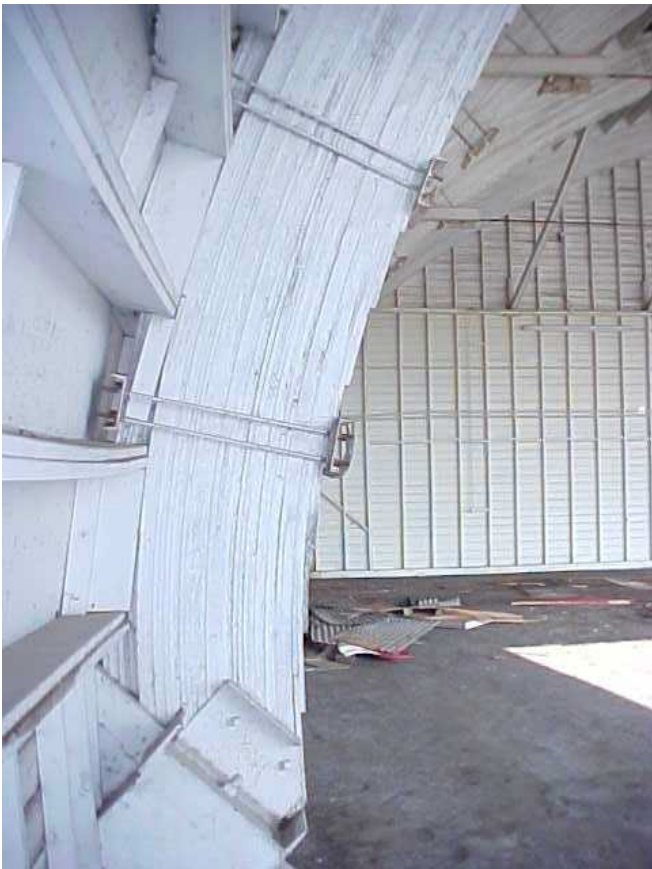
VIEWS OF WOOD LAMINATED ARCHES
