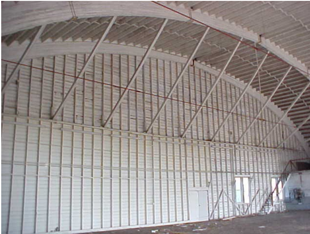
VIEW OF INTERIOR WESTERN WALL AND WOOD LAMINATED ARCHES
