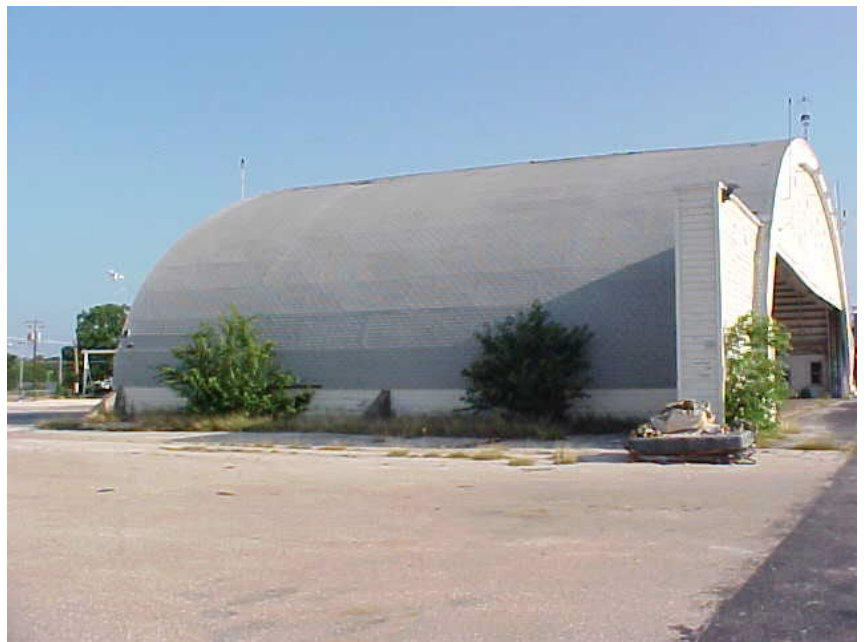
VIEW OF SOUTHERN FACADE WITH WINGWALL
