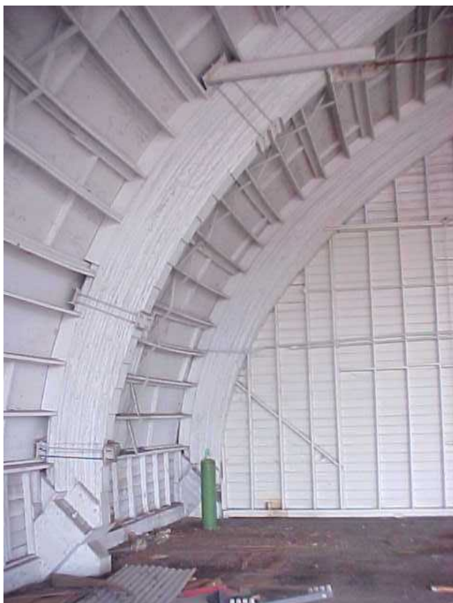
VIEWS OF WOOD LAMINATED ARCHES
