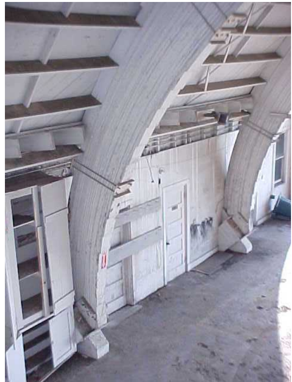
CLOSE-UP VIEW OF INTERIOR SHOWING ROOF SUPPORT SYSTEM
