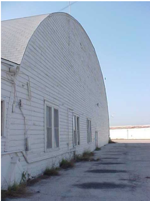
OVERALL VIEW OF AIRPORT BOULEVARD (WESTERN FACING) FACADE
