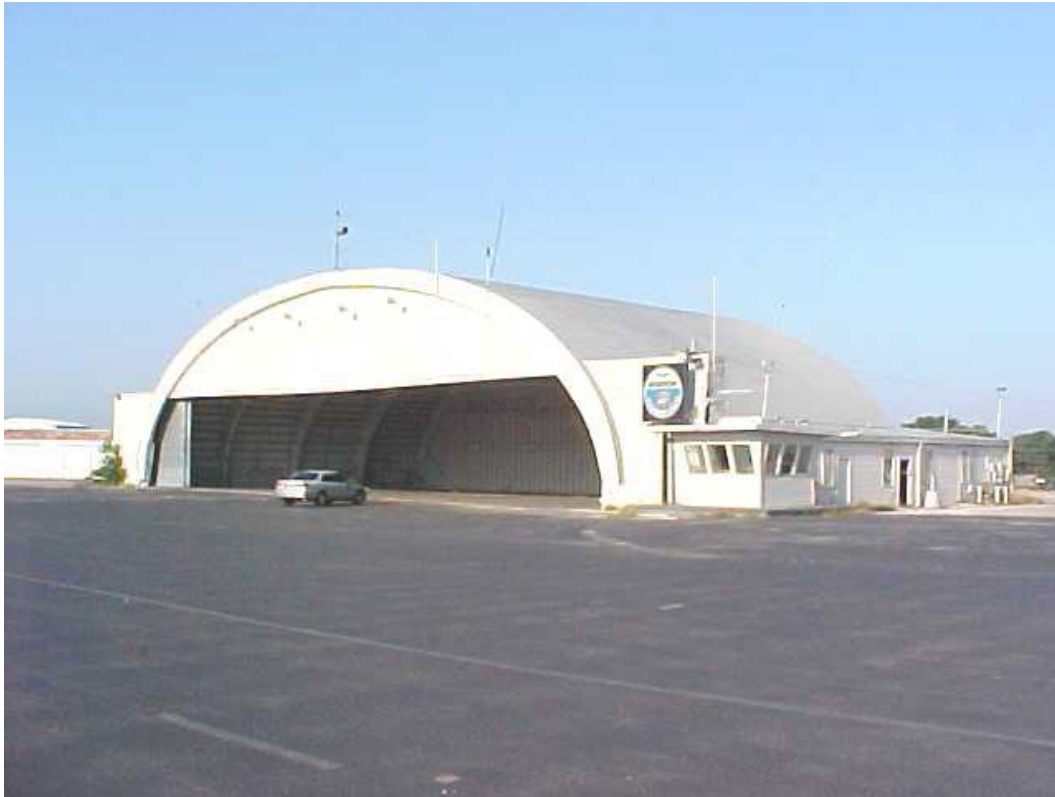
LOOKING WEST AT EASTERN FACADE OF HANGAR WITH DOORS OPEN
