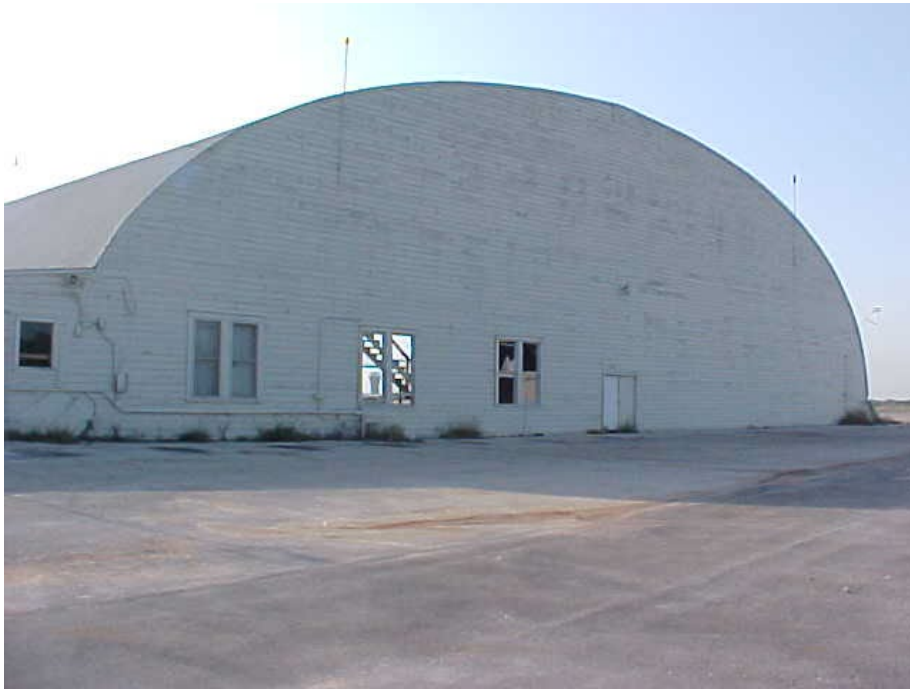
LOOKING EAST AT WESTERN FACADE (AIRPORT BOULEVARD FRONTING FACADE)
